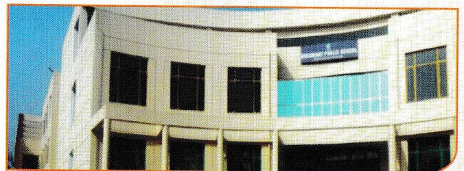
Bhagwant Public School, Chandpur (Bijnor)
